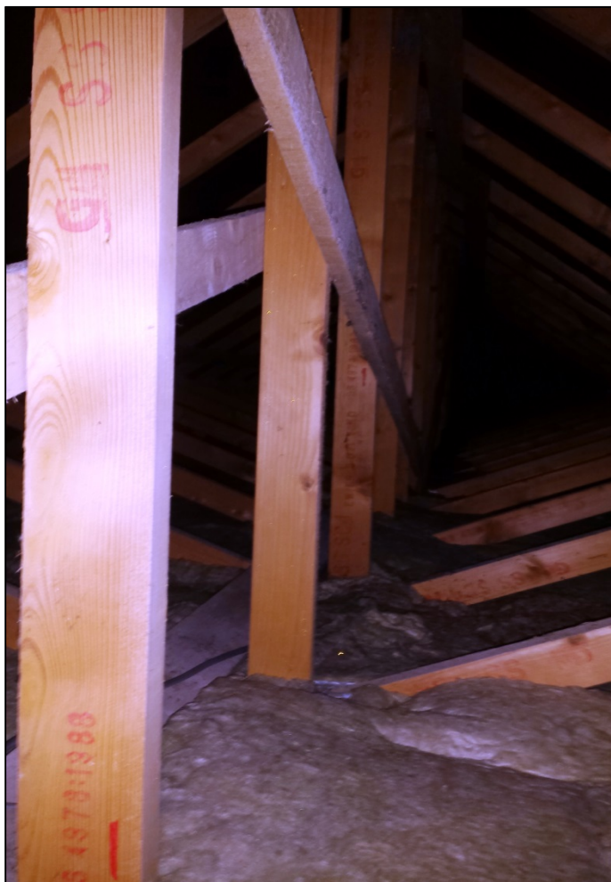
Plate 4 View of crawl space above Community Room
