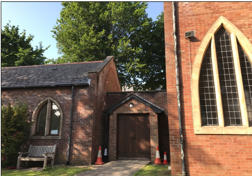
Plate 2 Community Room and flat-roofed connecting corridor to Nave
